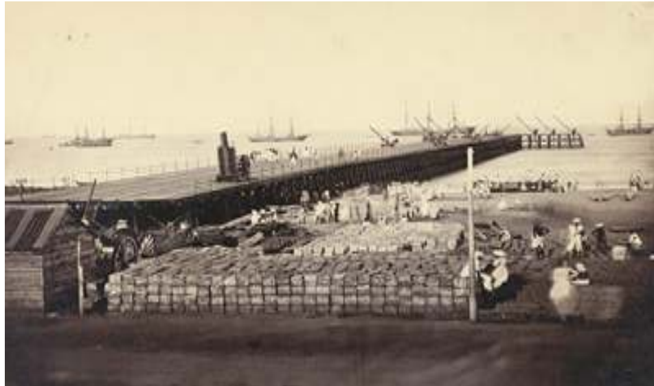
Photograph of the screw-pile pier under construction at Madras in c.1861.
