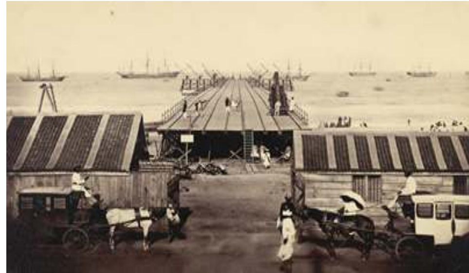
Photograph of the screw-pile pier under construction at Madras in c.1861.
