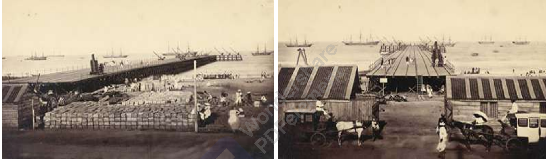
Photograph of the screw-pile pier under construction at Madras in c.1861.
