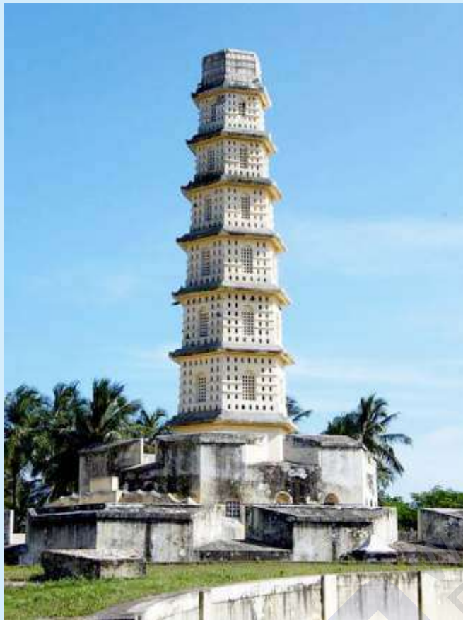
Manora was built by Thanjavur Maratha king Sarafojy - II in 1814 CE in Commomeration of victory of the British over Nepoleon. The hexagonal eight storeyed tower served as the light house also.
